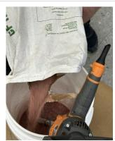
10. Slowly pour aggregate into the bucket. Using a variable speed drill and a Drywall Mud Mixing Blade, combine the aggregate and the liquid components.
