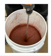
Continue mixing until all aggregate is wet out and no dry aggregate is observed.
