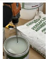
8. Using a variable speed drill and a Jiffy Mixing Blade, fully mix the Part A (Resin) and the Part B (Hardener).
