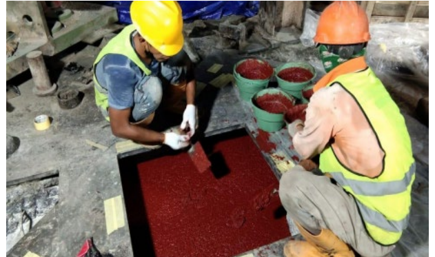
Installation of Chockfast Red into concrete foundation
