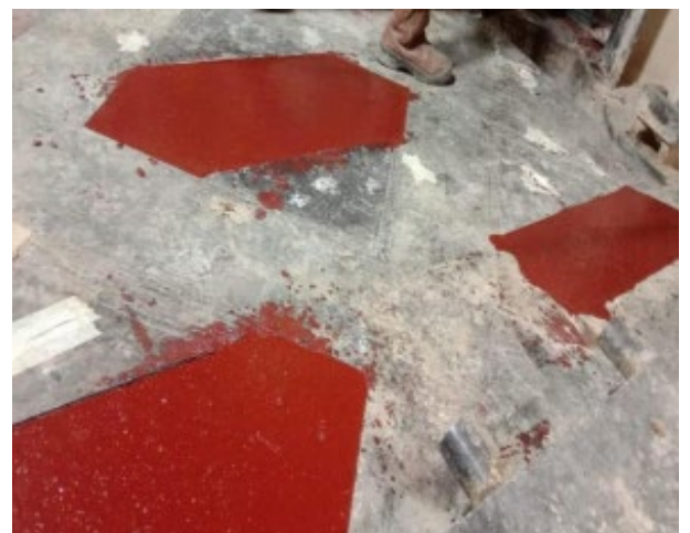
Cured Chockfast Red after installation
