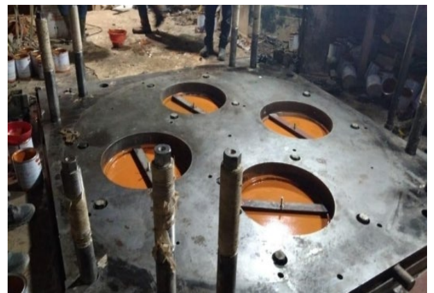
Chockfast Orange poured into raw mill machine plates
