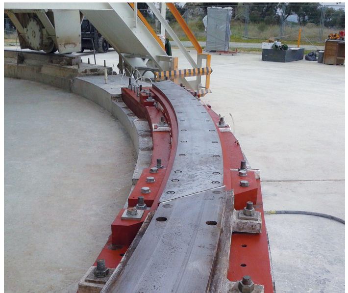
Completed repair of track with Chockfast Red
