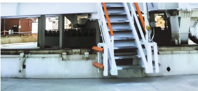
Damage along the concrete track
