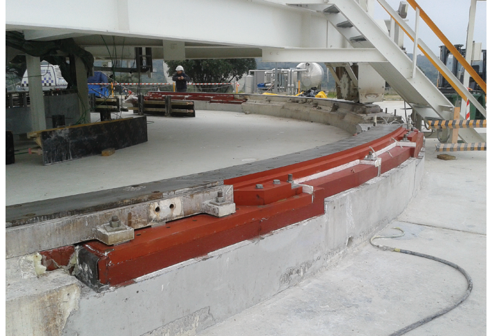
Side view of repaired track with Chockfast Red
