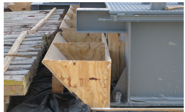
Headboxes constructed for effectively placing Chockfast Red
