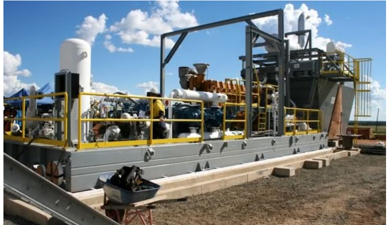
Compressor skid prior to placing Chockfast Red epoxy grout
