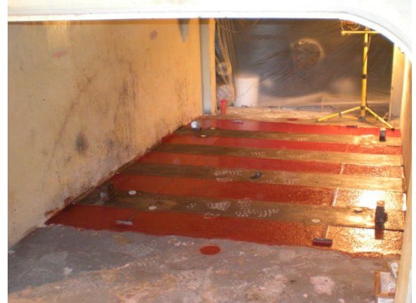
Chockfast Red poured into foundation forms
