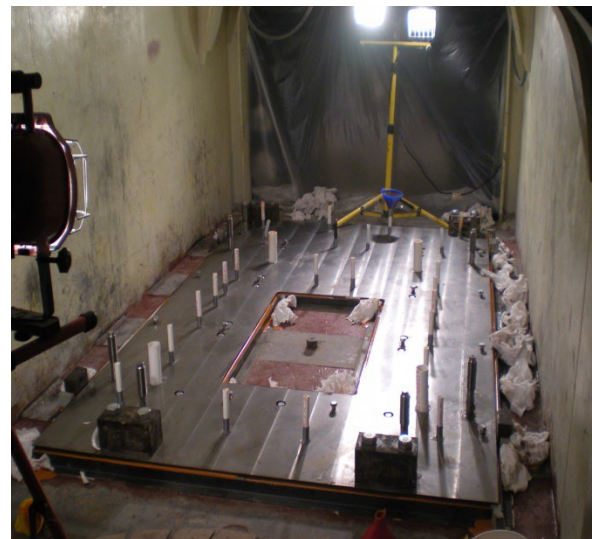
Base plate of the ball mill mounted
