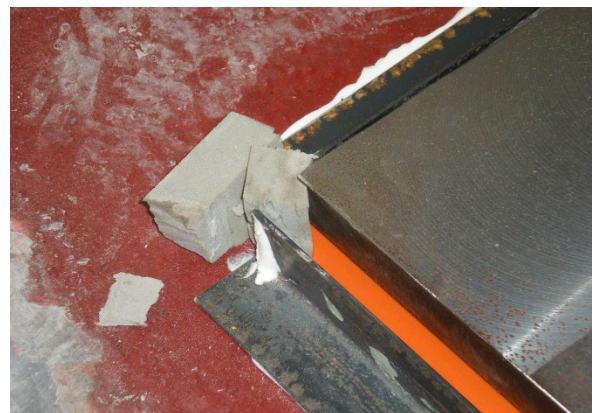
Closeup: Base plate of the ball mill mounted
