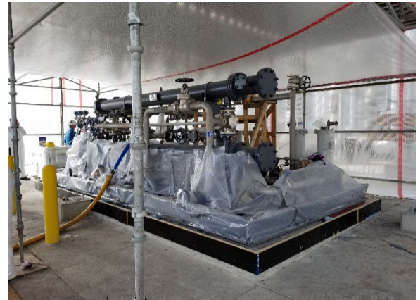
Lube oil skid formed and prepared for grouting
