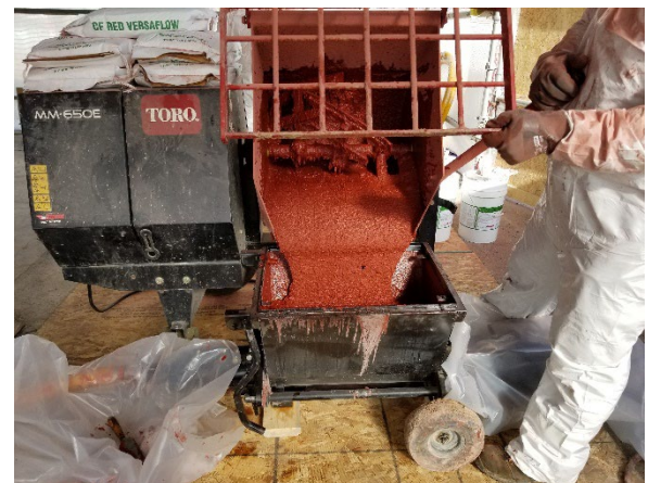
Dumping mixed Chockfast Red Versaflow into pump hopper
