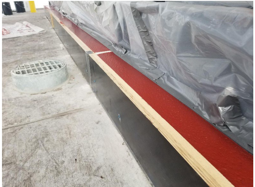
Cured Chockfast Red Versaflow under the lube skid
