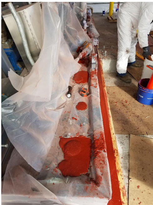
Chockfast Red Versaflow pumped into lube skid cavity
