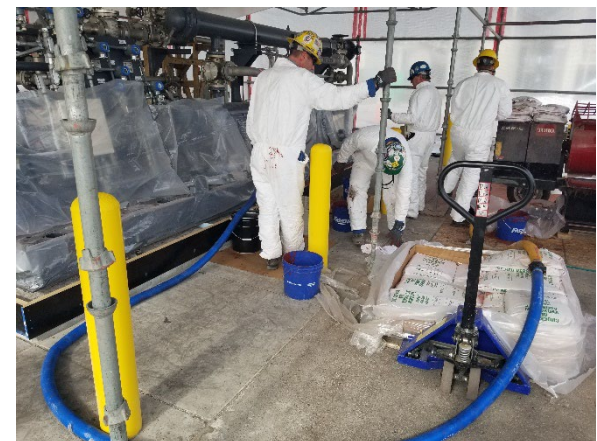
Chockfast Red Versaflow being pumped under the skid
