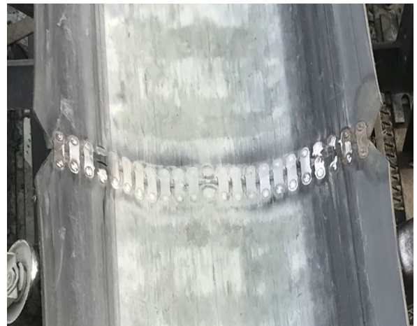
Corroded and abraded metal splicing
