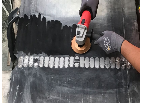
Abrading 8" with disc plate between metal splicing
