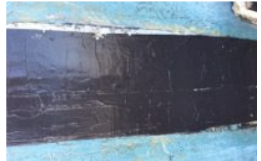
Devcon Flexane Putty applied to external tank
