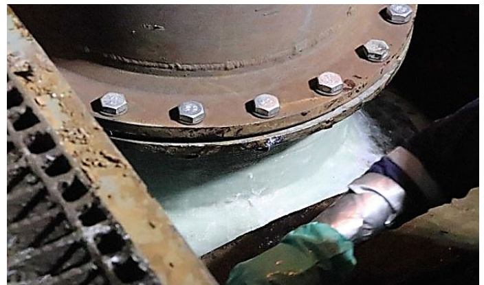
Repaired sea water outlet header back in service
