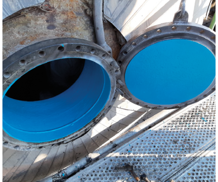
After being recoated with Devcon Brushable Ceramic Blue
