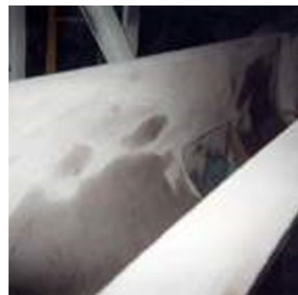
Trough after sand blasting and solvent application
