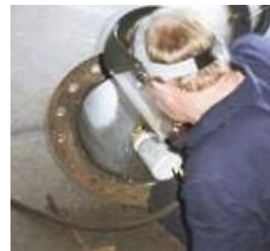
Devcon Combowear FC application to Pneumatic conveying pipe elbow
