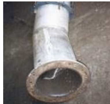
Pneumatic conveying pipe
