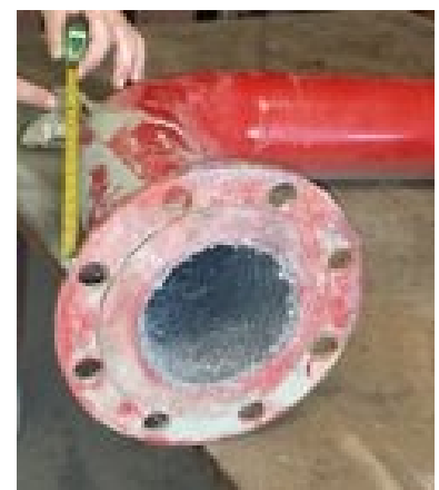
Pipe elbow coated with Devcon DFense Blok
