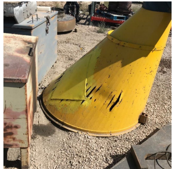
Steel AR plate tack welding to drill cone
