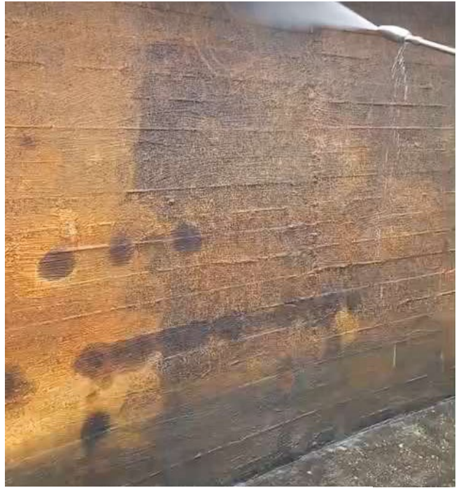
500 bar hydro surface preparation
