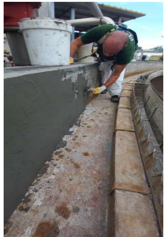
Concrete rebuild inside drainage channel with special cement
