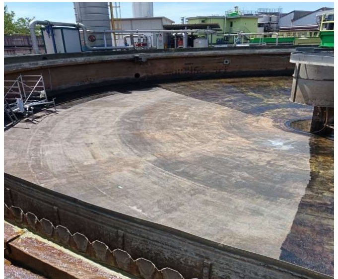
Coating of all internal surfaces with three coats of Devcon Epoxy Concrete Sealer
