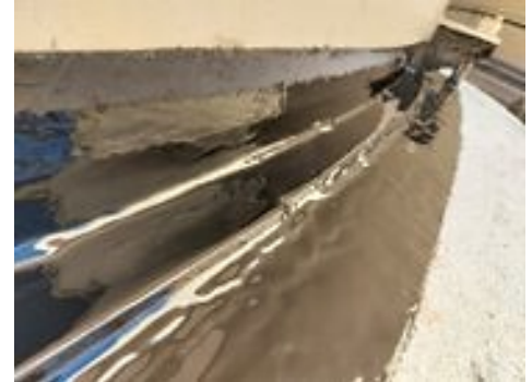
Full repair of holding tank foundation
