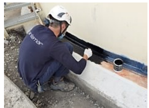
Devcon Flexane 80 Liquid application
