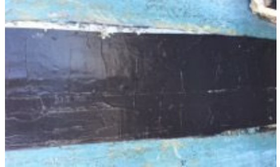
Devcon Flexane Putty applied to external tank
