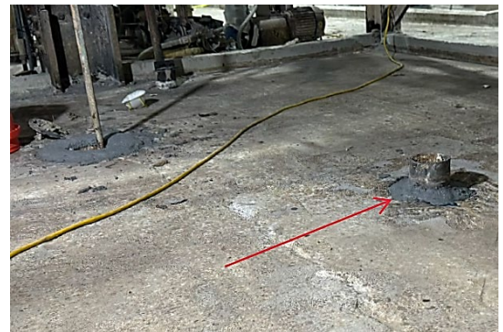
Devcon Floor Patch used around floor penetrations before pouring Devcon Floor Resurfacer
