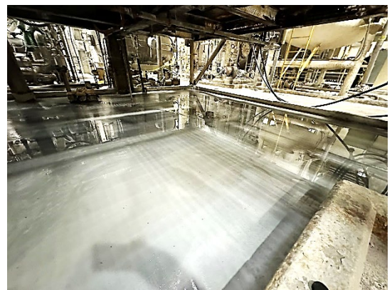
Devcon Floor Patch used around floor penetrations before pouring Devcon Floor Resurfacer
