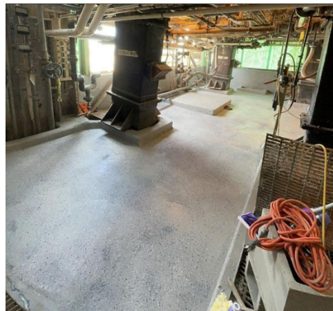
Slip-resistant paint covers the Devcon Floor Patch Resurfacer
