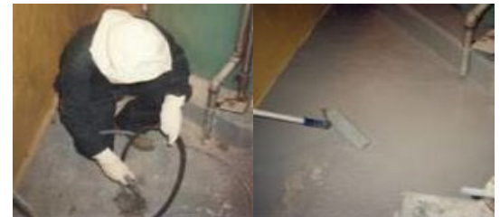
Sandblasting concrete floor & starting application
