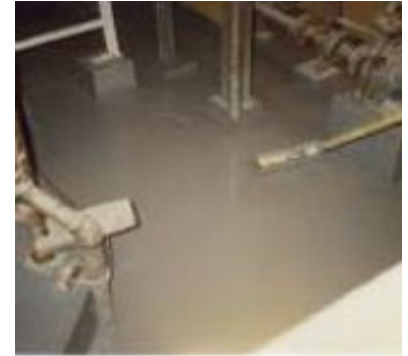
Concrete floor after Devcon Epoxy Coat 7000 AR and Devcon Epoxy Concrete Sealer
