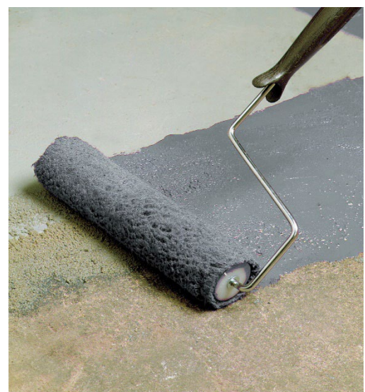
Devcon Epoxy Coat 7000 AR application to concrete flooring
