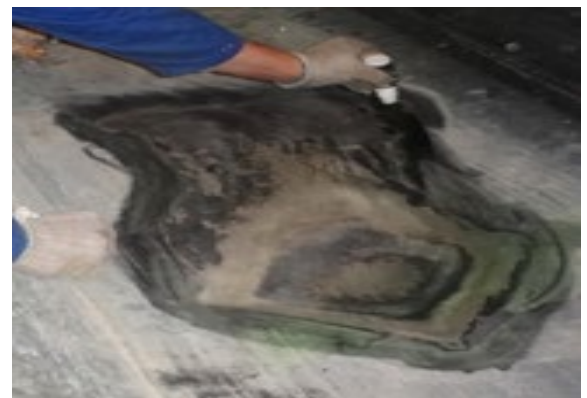
Damaged area of the transport belt
