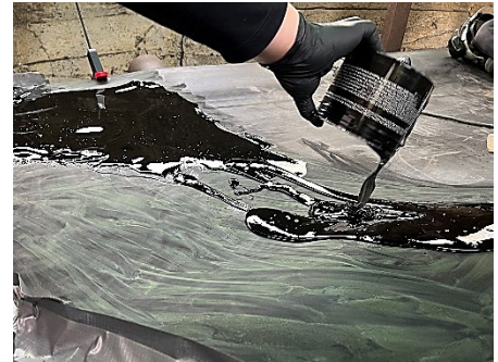
Applying Devcon R-Flex coating
