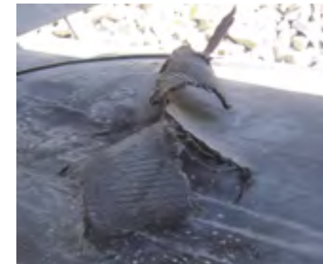
Before: R-Flex® Repair
