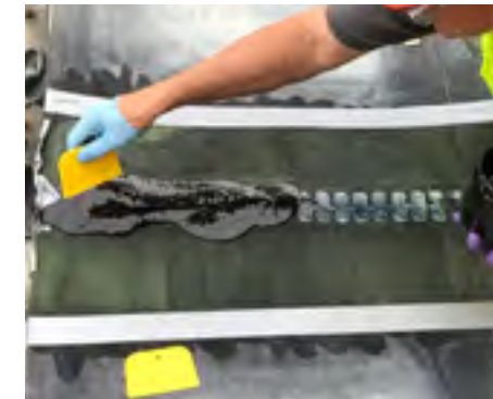
Before: R-Flex® Clip Repair
