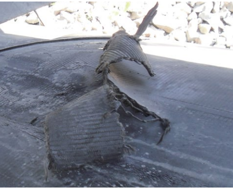
Before: R-Flex® Repair
