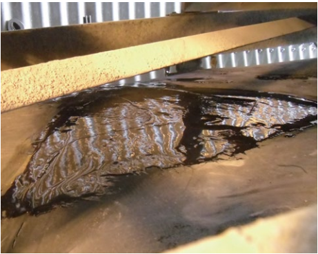
After: R-Flex® Repair Belt Running Strong
