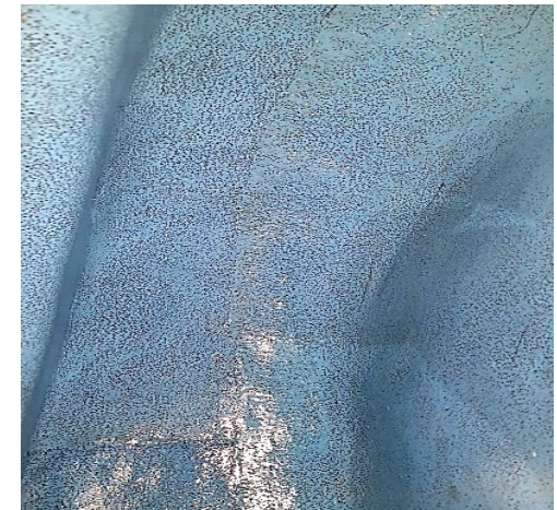
Devcon Wear Guard 300RTC extending into corners
