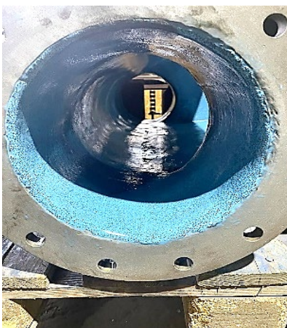
Devcon Wear Guard 300RTC applied to transfer chute interior
