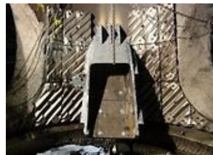
Vertical coal mill coal chute
