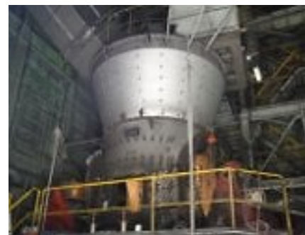
Vertical coal mill
