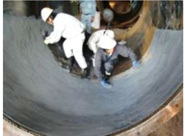
Application of Devcon Wear Guard Fine Load to coal dust collector
