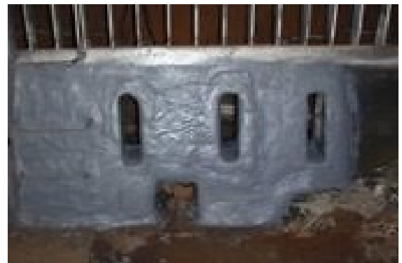
Drain face coated with Devcon Wear Guard Fine Load
