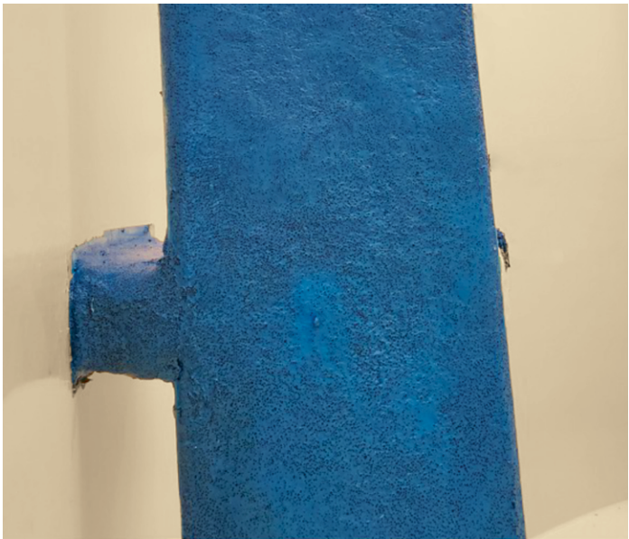
Devcon Wear Guard 300RTC Application Day 1
