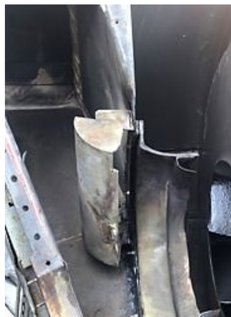
Leaking petrochemical exhaust flue
