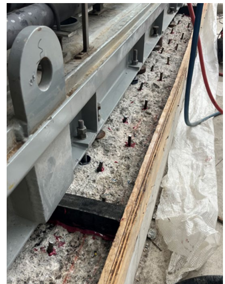
Figure 6: An example of Grout Pinning
