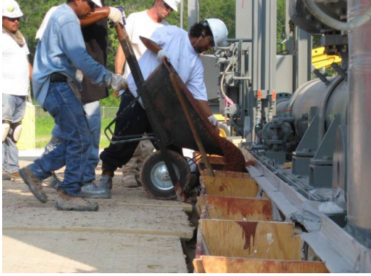
Figure 9: An example of using a Head Box to create head pressure
