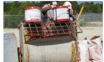
Figure 8: Example of a Horizontal-type Mortar Mixer
