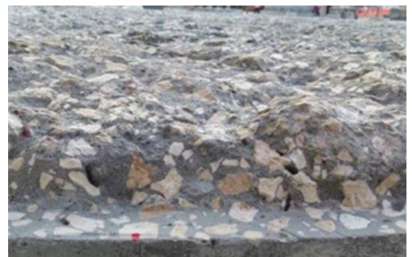
Figure 4: Example of Proper Concrete Surface Preparation
