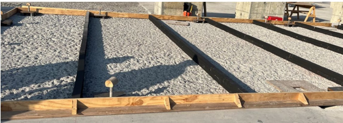
Figure 7: An example of a typical Expansion Joint Layout
