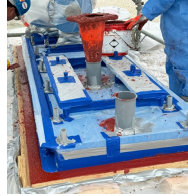
Figure 10: An example of using a cone to create head pressure
