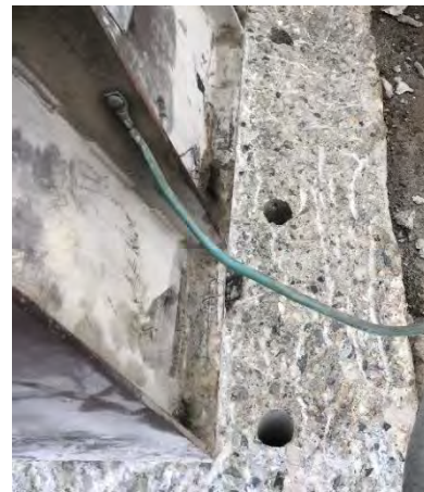
Figure 14: New Anchor Bolt Pockets in Properly Prepared Concrete Surface
