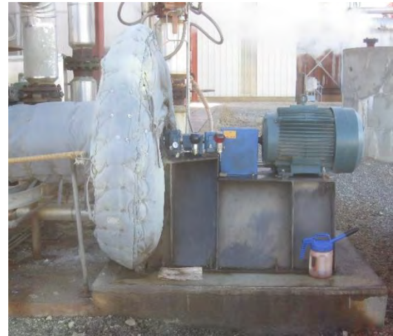
Figure 10: Original Equipment Installation
