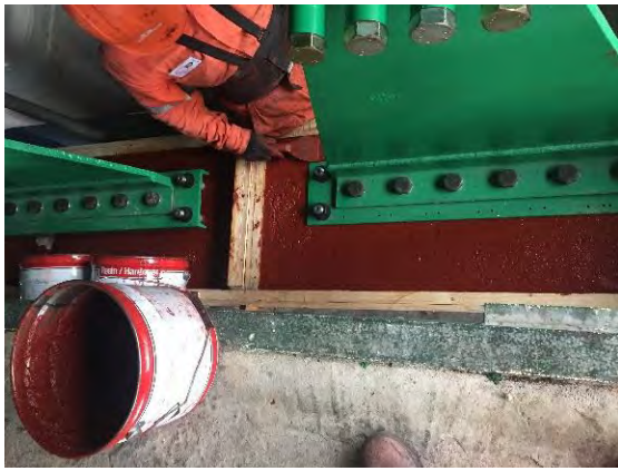
Figure 8: Superior Epoxy Grout Installed Under Compressor Support Rails
