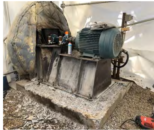
Figure 13: In-Process of Removal of Existing Epoxy Grout and Underlying Concrete
