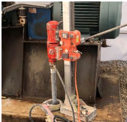
Figure 12: Core Drilling New Anchor Bolt Pockets
