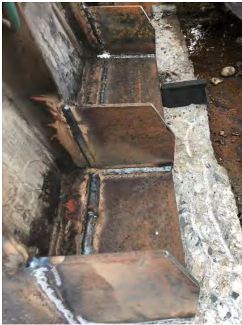
Figure 15: Baseplate Extension Welded to Existing Baseplate
