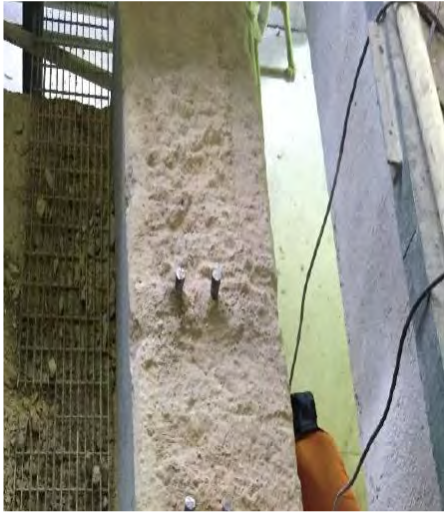
Figure 4: Surface of Concrete after removal of Cementitious Grout and Support Rails
