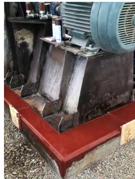
Figure 18: Final View of the Equipment Remediation
