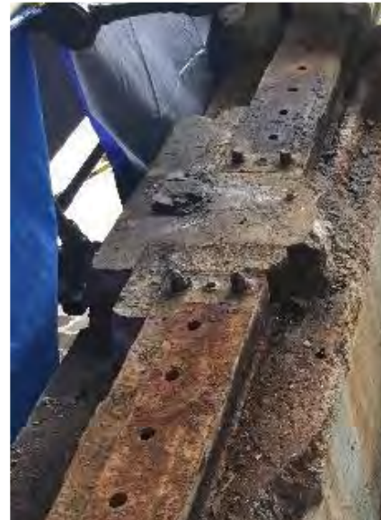
Figure 2: Removal of Existing Cementious Grout
