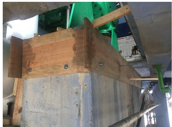
Figure 7: Formwork for Mounting Support Rails on Epoxy Grout
