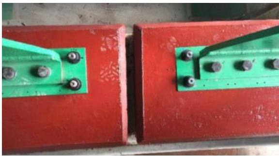
Figure 9: Final View of Compressor Support Rails on Superior Epoxy Grout
