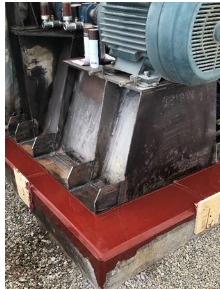
Figure 18: Final View of the Equipment Remediation
