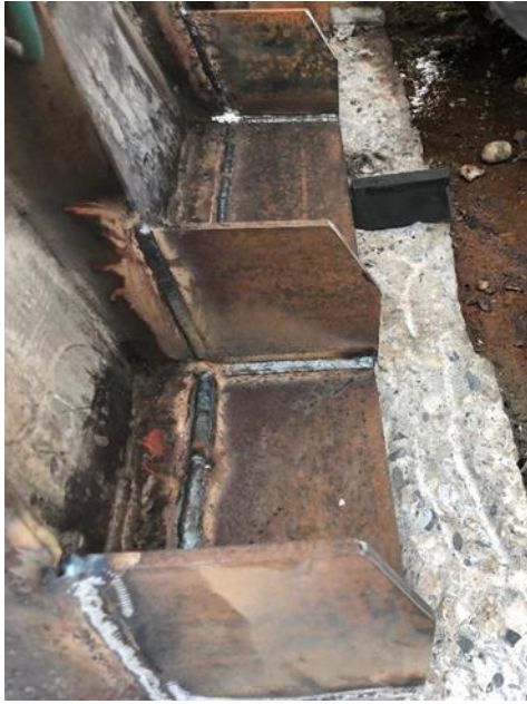
Figure 15: Baseplate Extension Welded to Existing Baseplate
