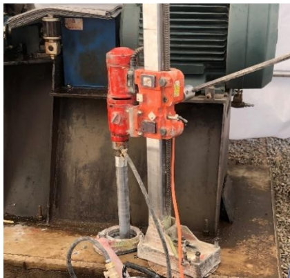
Figure 12: Core Drilling New Anchor Bolt Pockets
