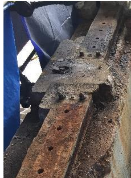
Figure 2: Removal of Existing Cementitious Grout
