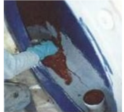
Brushable Ceramic Red applied to transfer pump
