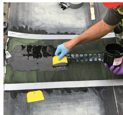
Before Metal Clips Splice Repair
