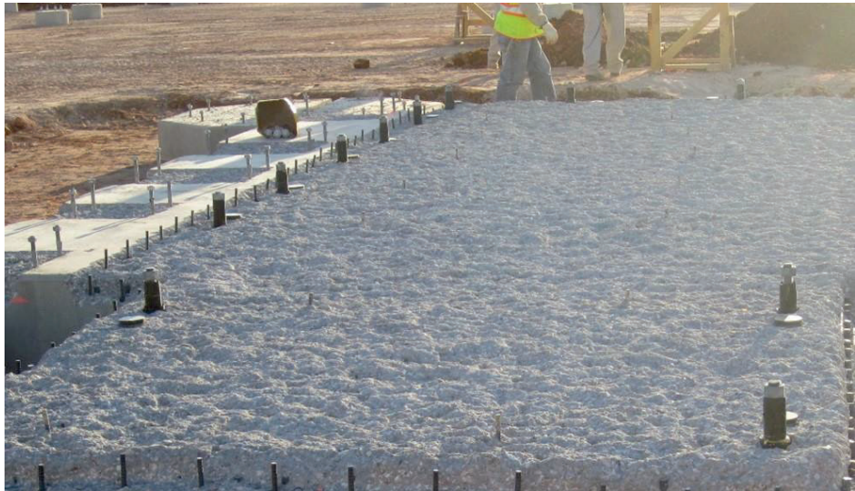
Figure 6: An example of a properly chipped foundation
