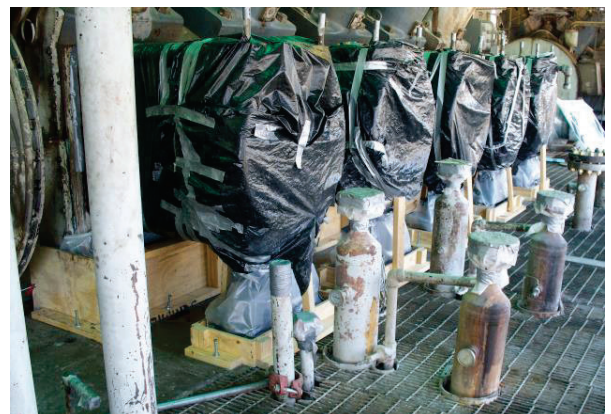
Figure 13: Installation of formwork
