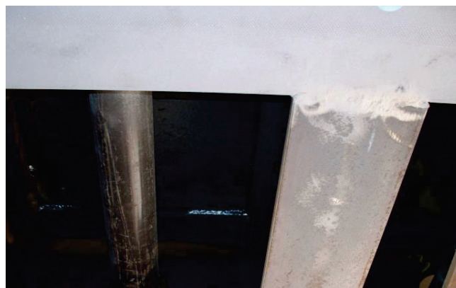
Figure 9: Abrasive blasted skid base flange
