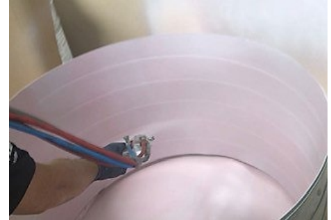
An example of spraying SprayCore AlphaCoat 1700
