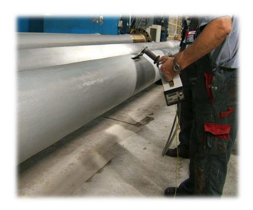
Mix the covering layer **WBD** resin and hardener to a homogenous mixture with our special mixer ...
