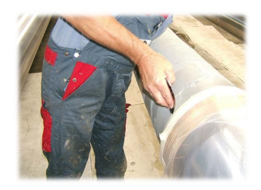
Measure the thickness with a magnetic thickness gauge after curing of **WBS** layer.
