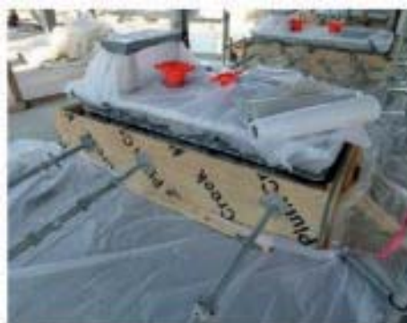
FIGURE 10 Braced grout form
