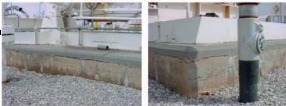
FIGURE 8 Temperature-induced cracks in concrete
